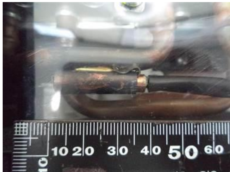
41. RAS-B10U2FVG-E,RAS-B10U2FVG-TR,RAS-B13U2FVG-E,RAS-B13U2FVG-TR, RAS-B18U2FVG-E,RAS-B18U2FVG-TR, thermistor
