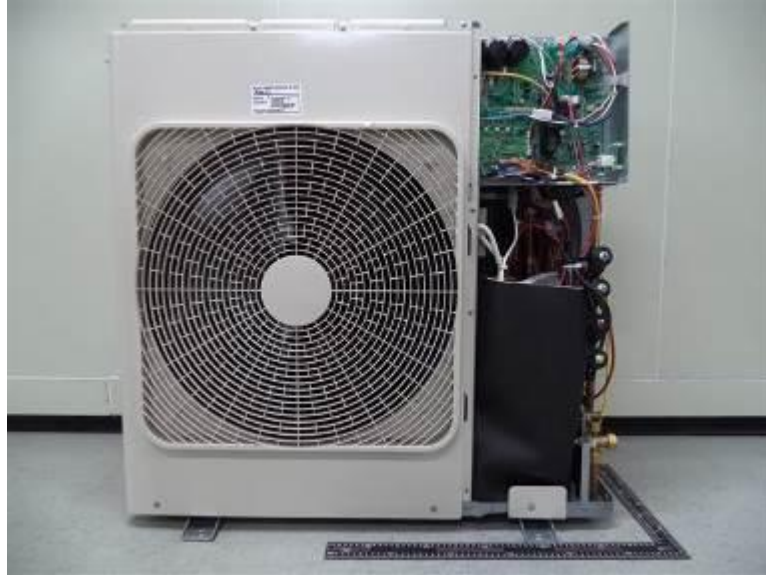
101. RAS-3M26U2AVG-E, RAS-3M26U2AVG-TR, RAS-4M27U2AVG-E, RAS-4M27U2AVG-TR, Internal construction
