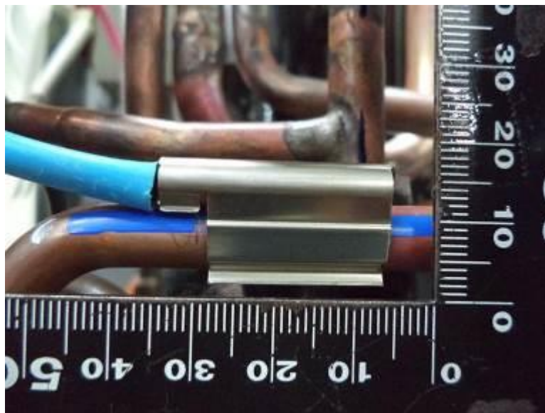
120. RAS-3M26U2AVG-E, RAS-3M26U2AVG-TR, RAS-4M27U2AVG-E, RAS-4M27U2AVG-TR, RAS-5M34U2AVG-E, RAS-5M34U2AVG-TR, Thermistor
