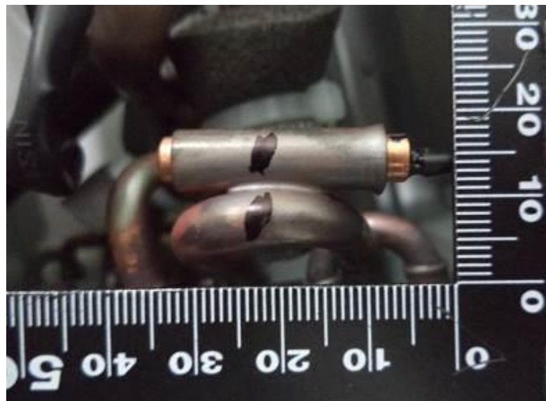
16. RAS-M07U2DVG-E,RAS-M07U2DVG-TR,RAS-M10U2DVG-E,RAS-M10U2DVG-TR, RAS-M13U2DVG-E,RAS-M13U2DVG-TR,RAS-M16U2DVG-E,RAS-M16U2DVG-TR, RAS-M22U2DVG-E,RAS-M22U2DVG-TR,RAS-M24U2DVG-E,RAS-M24U2DVG-TR, coil sensor
