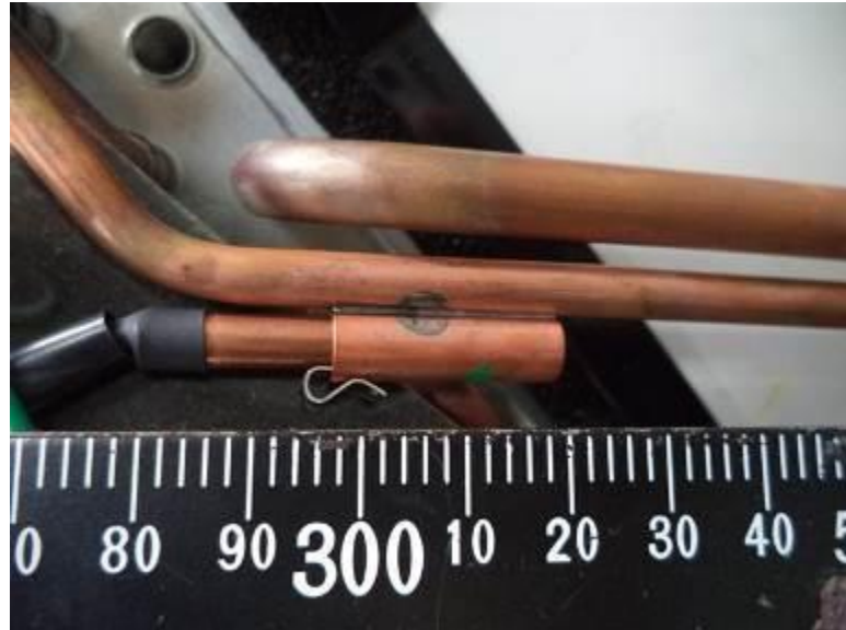
40. RAS-B10U2FVG-E,RAS-B10U2FVG-TR,RAS-B13U2FVG-E,RAS-B13U2FVG-TR, RAS-B18U2FVG-E,RAS-B18U2FVG-TR, thermistor
