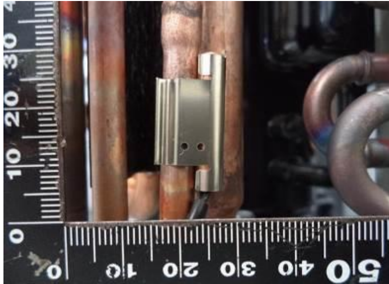
117. RAS-3M26U2AVG-E, RAS-3M26U2AVG-TR, RAS-4M27U2AVG-E, RAS-4M27U2AVG-TR, RAS-5M34U2AVG-E, RAS-5M34U2AVG-TR, Thermistor
