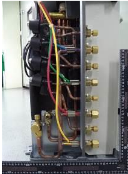
109. RAS-3M26U2AVG-E, RAS-3M26U2AVG-TR, RAS-4M27U2AVG-E, RAS-4M27U2AVG-TR, Refrigerant connection
