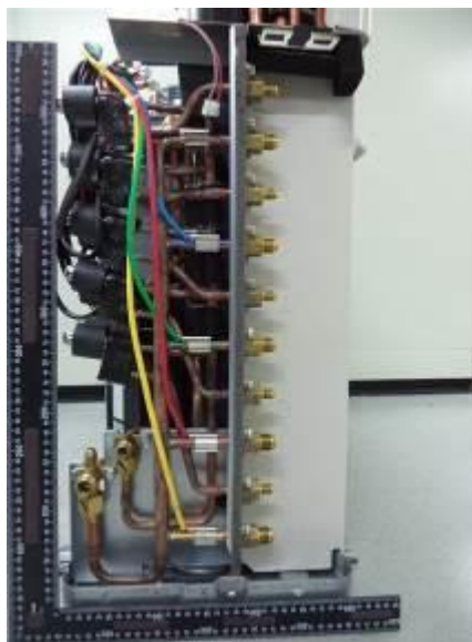
110. RAS-5M34U2AVG-E, RAS-5M34U2AVG-TR, Refrigerant connection
