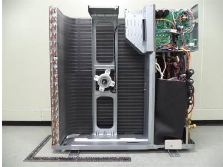
105. RAS-3M26U2AVG-E, RAS-3M26U2AVG-TR, RAS-4M27U2AVG-E, RAS-4M27U2AVG-TR, Internal view removed fan blade
